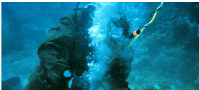
Fig. 26. A diver uses an underwater pneumatic drill to prepare the substrate at a receiving site for attachment of relocated coral colonies. Such an approach can provide cavities for epoxy or cement to allow a better ‘grip’, since biofilms on natural substrates often result in poor adhesion. Source: Erik Zobrist (CCO-PD).
