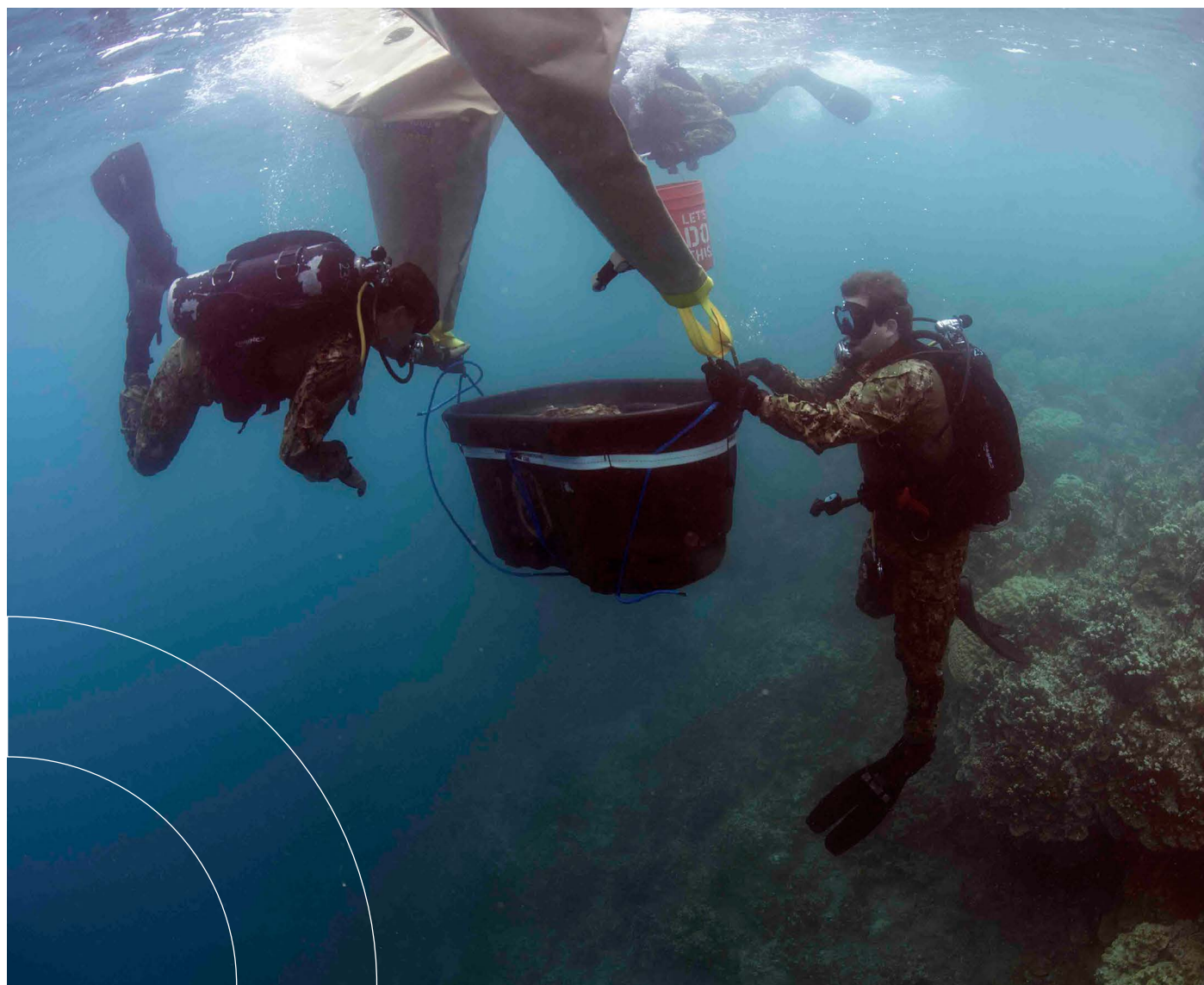
Fig. 24. Technicians use lift bags and crates to relocate large coral colonies. Such an approach reduces handling stress and limits air exposure time. Source: Alfred A. Coffield (CC-BY-NC-ND 2.0).
